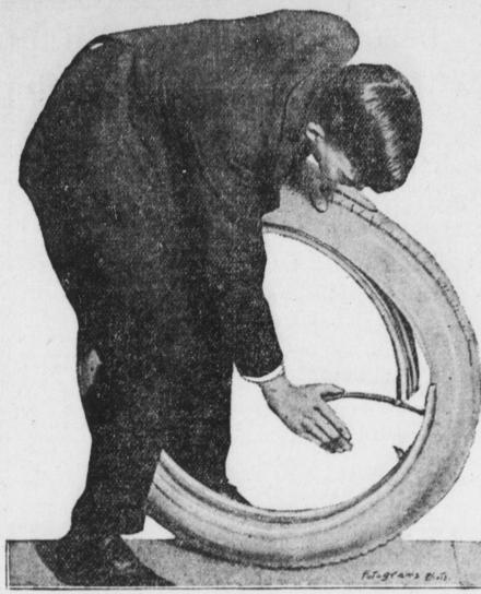
As a result of the incessant annoyance, loss of time, and general inconvenience which the motorist suffers when a change of tires becomes necessary. inventive genius has frequently been directed toward the elimination of tirechanging troubles. A new device, called the Lever-Lock, is applicable to any type of standard rim, and permits of a tire change in the speedy time of one minute. It is simple to operate and effective.
