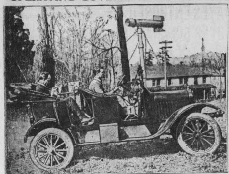
W. S. James and C. S. Bruce of the automobile power plant of the insean of standards, driving the test car used to determine the power output of the engine, combustion valve of the fuel, wind resistance, etc. This car is wise used in experiments to discover gasoline substitutes and is fitted with a gramera which automatically records the fuel consumption.
