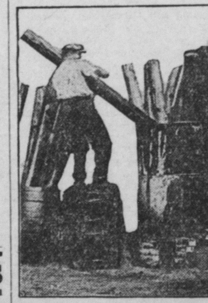
Removing posts After treatment in Creosote—The Posts Are Allowed to Drain in the Barrels.
