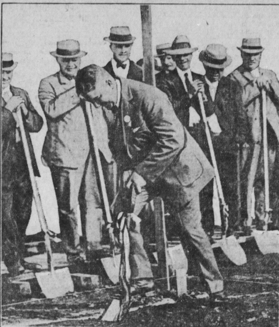
The photograph shows Gov. Harry L. Davis turning the first spadeful of earth at the ground-breaking ceremonies of the new Ohio stadium, to be erected at a cost of $1,341,017, on the campus of Ohio State university at Columbus, Ohio.
