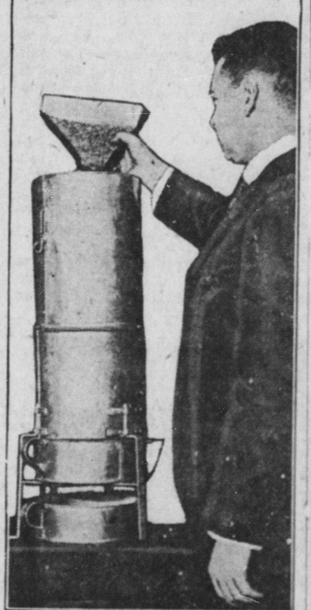
Pouring a Sample of Grain into a "Modified Boerner Sampler."
