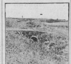
Method of Carrying Terrace Water Under'a Roadway by Means of a Cul-
