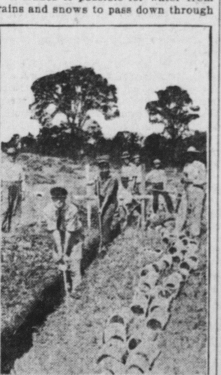
Students Constructing Tile Drain.
