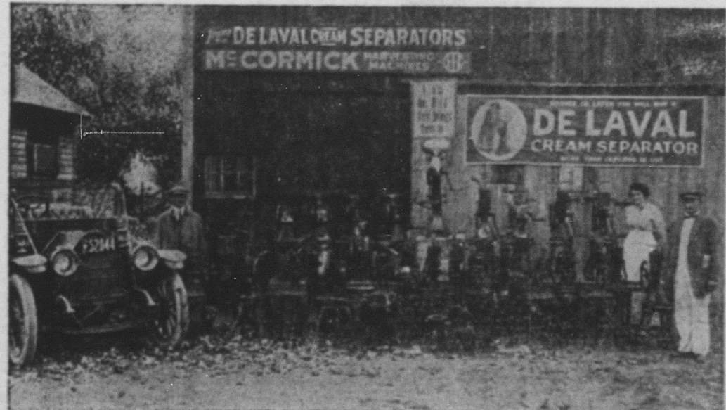
This imposing array of inferior and worn-out machines were taken in trades for cream saving De Lvals in a period of a little over two months by D. W. Bradford, De Laval Agent at Centre Hall, Pa.
