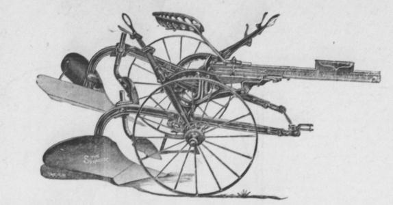
It plows the same depth the wholesday long ; sticks to the ground in stormy soil ; can be well handled on rocky hillsides. It leaves no deep furrows to wash ; will throw the soil up hill better than any other plow made ; it is strong enough to do its work, yet not clumsy. Made for two or three horses.
