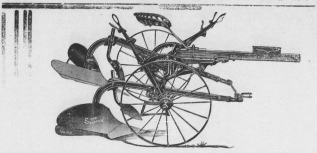
It plows the same depth the whole day long ; sticks to the ground in stormy soil ; can be well handled on rocky hillsides. It leaves no deep furrows to wash ; will throw the soil up hill better than any other plow made ; it is strong enough to do its work, yet not clumsy. Made for two or three horses.
