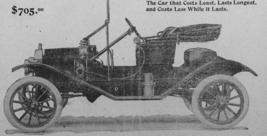
This Car delivered to you with full equipment, including top, wind shield, speedometer, three oil lamps, gas lamps, and generator, tools and tire repair kit, for \$705.00.
