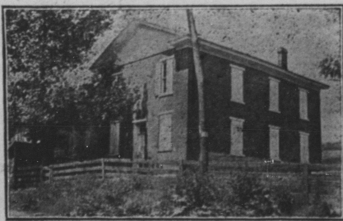
OLD BUILDING AT PENN HALL, ERRECTED 1866.
