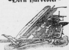
Reciprocating feeding jaws reach well ahead of the knife and force the cut. Will not pull corn up by the roots.
