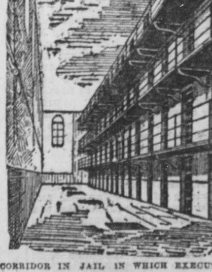
CORRIDOR IN JAIL IN WHICH EXECUTION TOOK PLACE.
