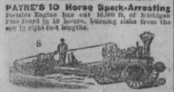
Our 10 Horze We Guarantee to furnish power o saw 8,000 feet of Hemlock boards in 10 hours. fur 15 Horse will cut 10,000 feet in same time. Our Engines are guamantees to furnish a horse-power on i, loss fuel and water than any other Engine not fitted with an Automatic Cut-Off.
