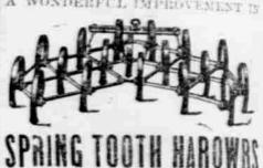
Teeth Quickly Adjusted Loosening One Nut
