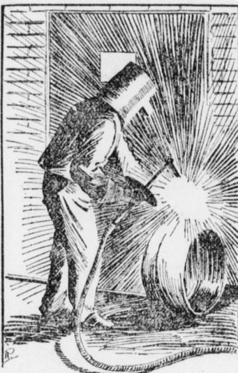
The Benardos Process in Use.
