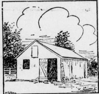
The Shelter That Housed 36 Hogs.
