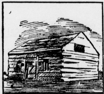
Old Church as it Appeared Before Its Restoration.
