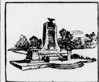
MONUMENT BEING ERRECTED AT ANDERSONVILLE, GA.
