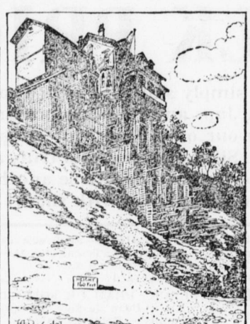
LIFTED ONE HUNDRED FEET.
