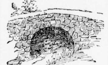
ROUGH STONE CULVERT.
