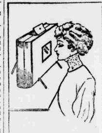
can be adjusted to any position desired, the magnifying glass in the front enlarging the views and bringght, supplied from the battery in the storage compartment, illumines the exhibition chamber and enhances the general effect of the picture. For evenings at home this device can be made both instructive and entertaining with a collection of historic views.
