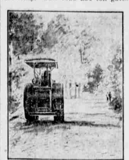
MODERN ROAD MAKING. (Preparing Government Sample Road at Hot Springs, Va.)
