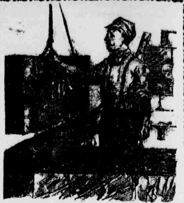
"A Good Foundation."
