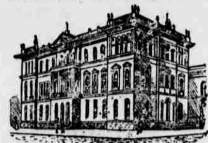
A CRUMBLING STRUCTURE. In the court room many noted criminals have been tried, and in the annexed jail and jail yard some of the worst have taken the drop for eternity.
