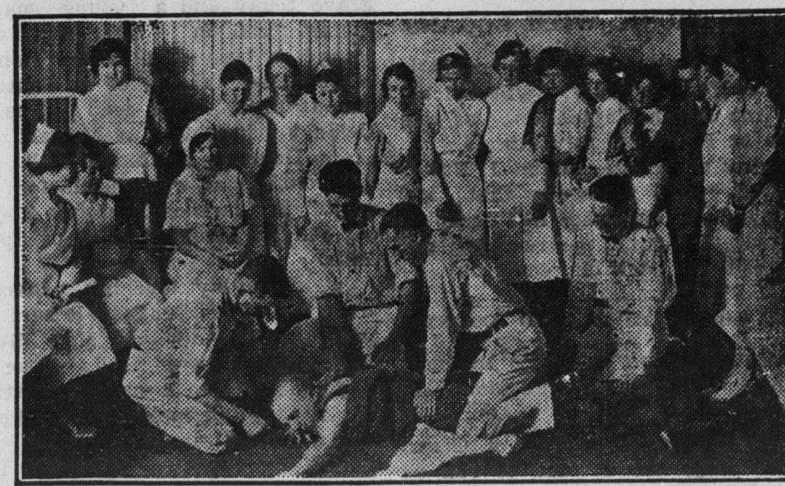
Nurses of the graduating class of the Pittsburgh Presbyterian Hospital displayed keen interest recently in a special first aid demonstration by the Bell Telephone Company of Pennsylvania. Members of the company's construction department are skilled in first aid methods, and frequently have occasion to render some form of public service in emergencies.
