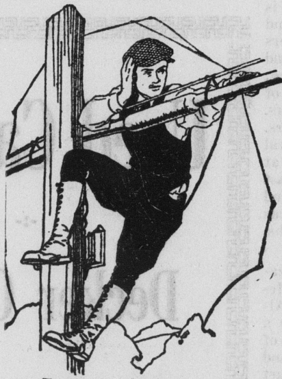
Testing Aerial Cable
