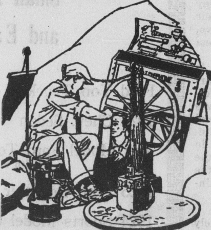
Working on Underground Cable
