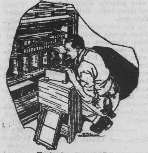
Working in a Central Office
