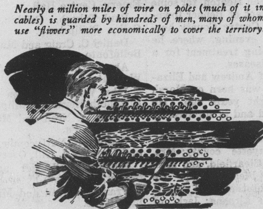
Inside the Bell Buildings, "central office men" are always on duty, making tests, checking up, and watching the millions of connections, every one of which must be perfect.
