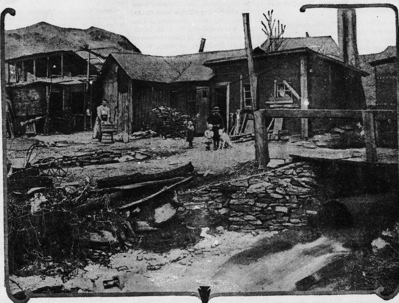
This is not the picture of a sewer. It is the supply pipe which carries the water supply of a city of eleven thousand inhabitants.
