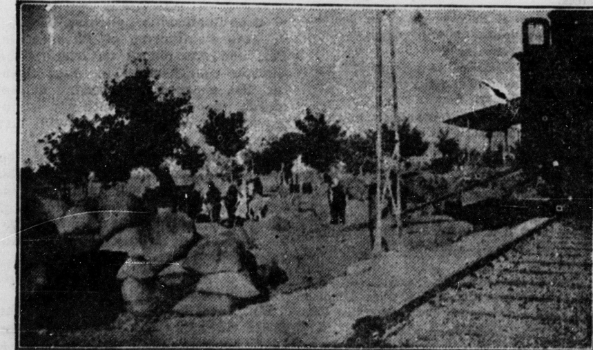
Shoveling Grain on the Line of the Bagdad Railway.
