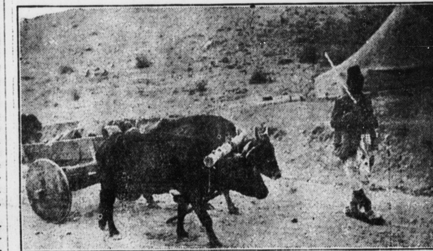
Building the Hejaz Railroad.
