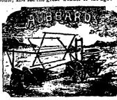
COMBINED MACHINE weighs only eight hundred pounds. Delivered free of freight this year only. Steel finger-bar with folding joint. Flexible apring steel draft bar. Adjustable effiptic spring sest Adjustable grain-divider.
