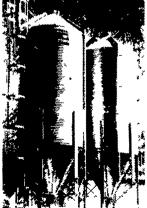
n in High Capacity 40° roof (left) allows more storage and stays cleaner than ntional 30° roof (right)
