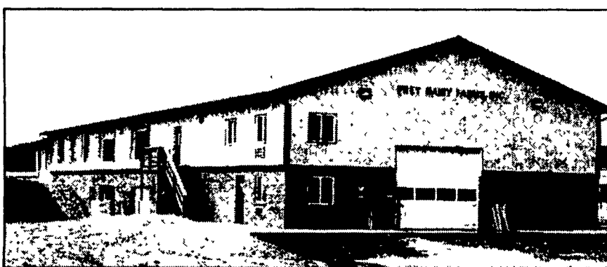
Frey Dairy Farms Complete Dairy Complex Conestoga, PA (Lancaster County)
