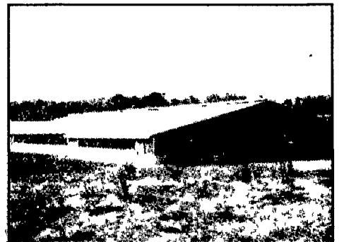
Free Stall Barn Exterior
