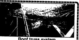
Roof truss system 50 wood trusses that are a single slant. 50' long... also galvanized roofing.
