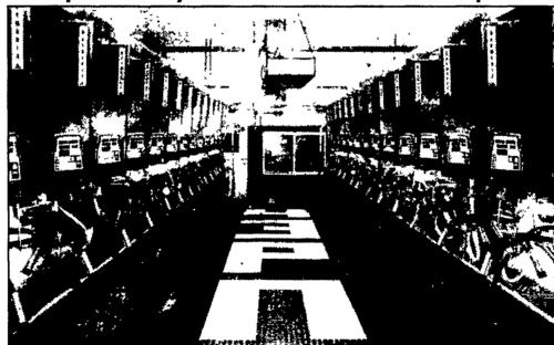
Lauden Farm was retrofitted from a double 5 tandem parlor to the new Germania double 16 all stainless steel fastback stalls. The parlor was installed between milkings.
