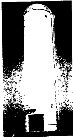
POURED CONCRETE SILOS
