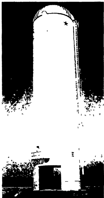
POURED CONCRETE SILOS
