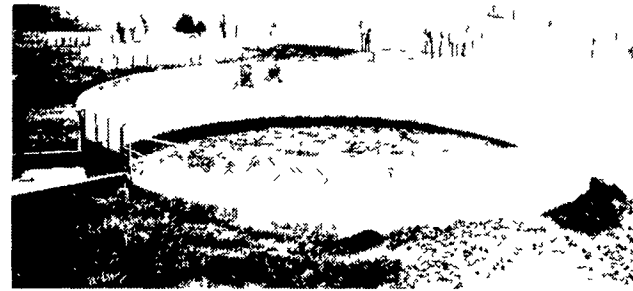
CONCRETE TANKS: PRECAST OR POURED IN PLACE: NRCS CONCURRED. ABOVE GROUND OR BACKFILLED.
