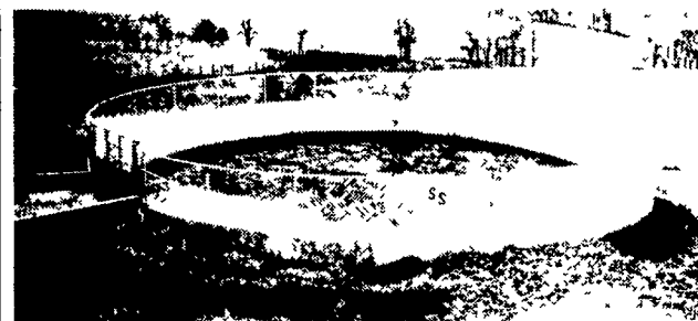
CONCRETE TANKS: PRECAST OR POURED IN PLACE: NRCS CONCURRED. ABOVE GROUND OR BACKFILLED.
