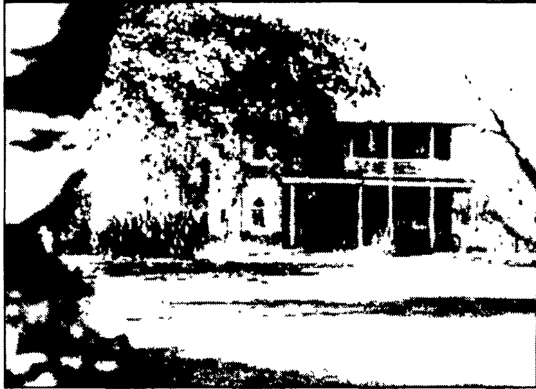
Salvaged materials were used to restore this house.
