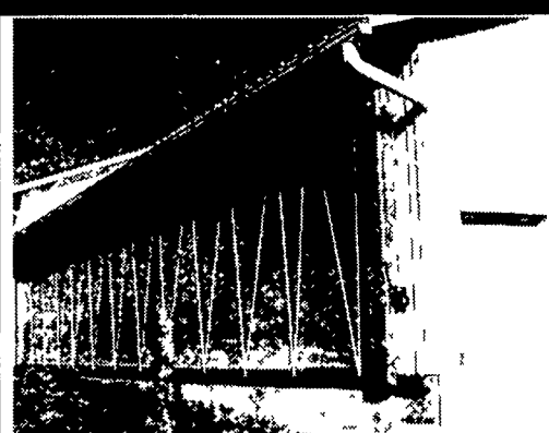
Delta, PA 8'x48' Installation
