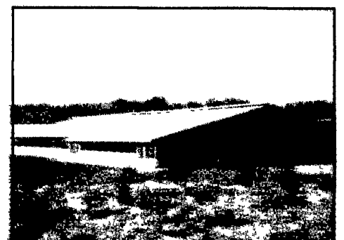
Free Stall Barn Exterior
