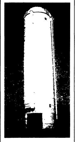
For Maximum Convenience: **Poured Concrete Silo with** Drive Thru Tunnel and the Big Jim Quantum Unloader.
