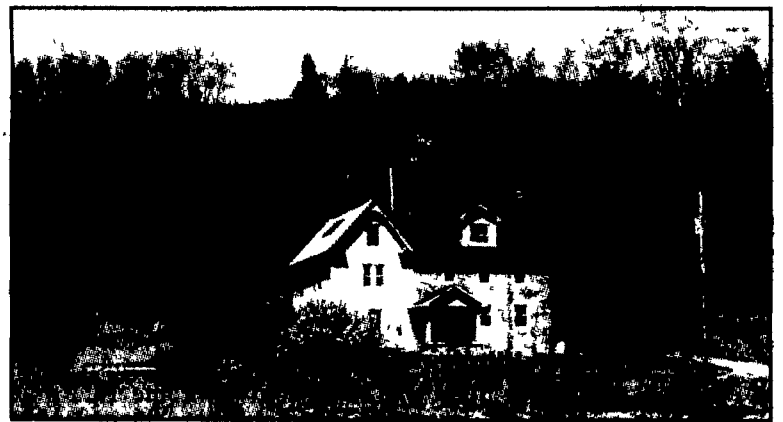
The renovated 1820 farm house at Cedar Hill at Spruce Creek Bed and Breakfast is surrounded by breath-taking views guests can savor year-round.
