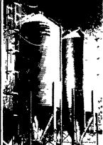
عد تعدا High Capacity 40° roof (left) allows more storage and stavs cleaner than entional 30° roof (right
