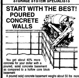
A poured solid concrete basement weighs about 50 lbs more per cubic foot! Far denser. What's more, poured solid concrete walls are monolithic . . there are no joints!
