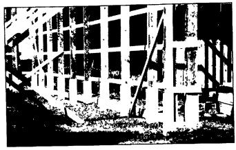
Protector prevents underground wooden posts, used in post frame construction, from rotting or being destroyed by insects.
