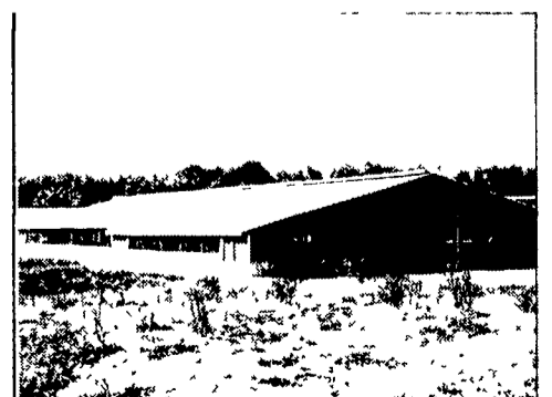
Free Stall Barn Exterior
